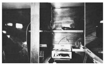
**Figure 26-8** *Rogue Wave's* galley area after the deck was installed. Sandwich construction of the deck in this area required a headliner skin. This smooth plywood panel was painted white to lighten the naturally finished interior.
