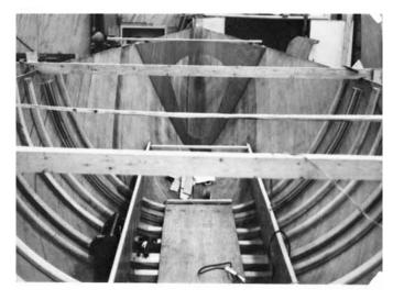
Figure 11-8 Laminated frames fit to a hull.
