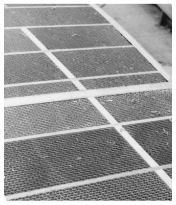
**Figure 27-25** A sandwich deck with all of the framing and honeycomb core in place before the top plywood deck surface was laid.
