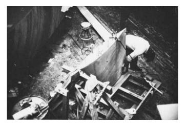
**Figure 14-23** A keel set up in a specially-built handling fixture so it can be final faired and moved around.
