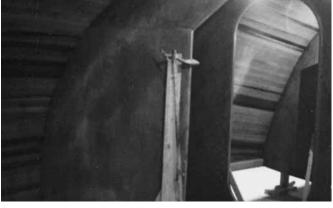
**Figure 23-10** The 42' hull with the temporary mold removed. The hull is supported by permanent bulkheads installed during set-up. Note the clean interior in which work can progress while exterior finishing is completed.
