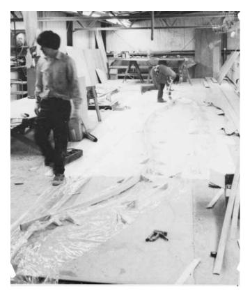
**Figure 11-2** Laminating a long structural member for trimaran crossbeam using cleats secured to the lofting floor.
