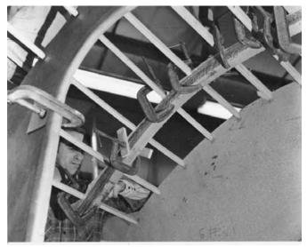
**Figure 11-4** Laminating floor timbers using stringers as the form.
