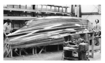
**Figure 15-1** Coating the exterior of an IOR ½-ton racer. This boat has a natural finish. All fairing, finish sanding, and coating were done prior to removing the hull from the mold.
