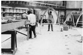
Figure 18-4 Setting up the first frame.
