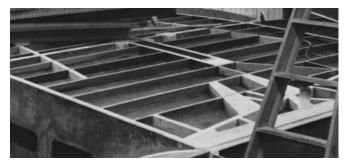
**Figure 27-23** Sawn Sitka spruce blocking is bonded to core deck at all structural frames and planed flush with the deck profile. Note the strip of blocking for adjustable sail leads to the left.
