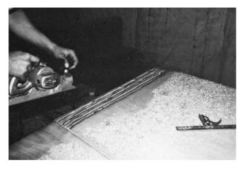
**Figure 12-10** Use a power plane to rough shape a scarf bevel. Finish shaping the bevel with a block plane.
