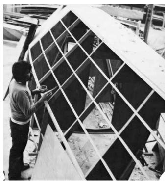
**Figure 24-8** Applying adhesive mixture before bonding a panel to the framework. The panel lying against the framework in the foreground will be scarfed in place.
