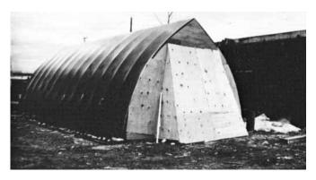
**Figure 8-18** Shelter completed. Plywood walls were used at both ends to give the structure extra rigidity.
